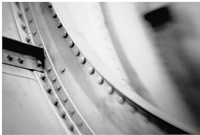
Typical riveted panel and stiffener
